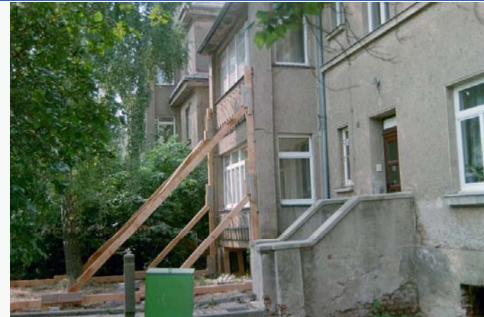
D3: Subsidence, cracks
